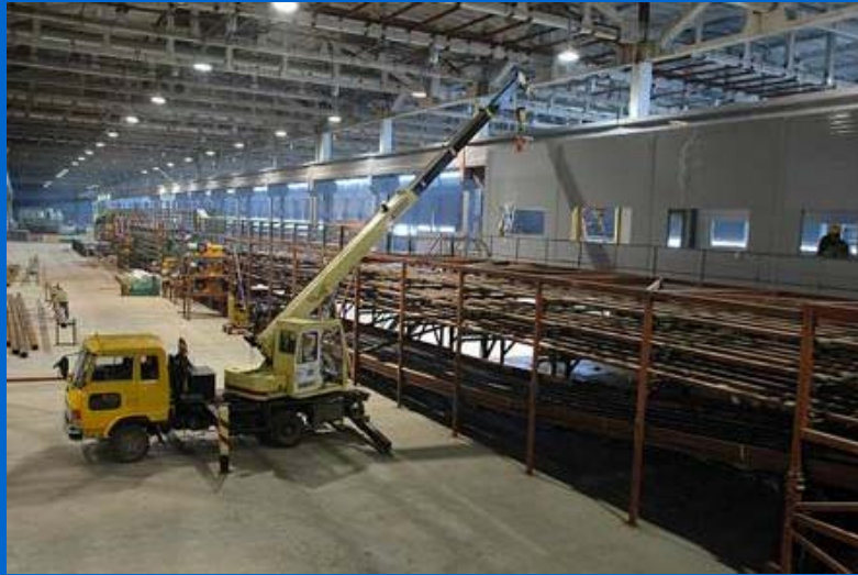
Construction of the peeling line control room, September 8, 2010.
