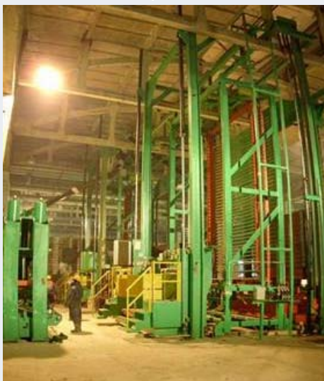
Press Installation Begins At The Sosnovoborsk Mill. Photo Taken On February 12, 2010.
